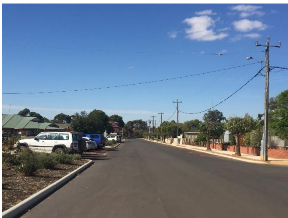
Whittington Street - easterly view
