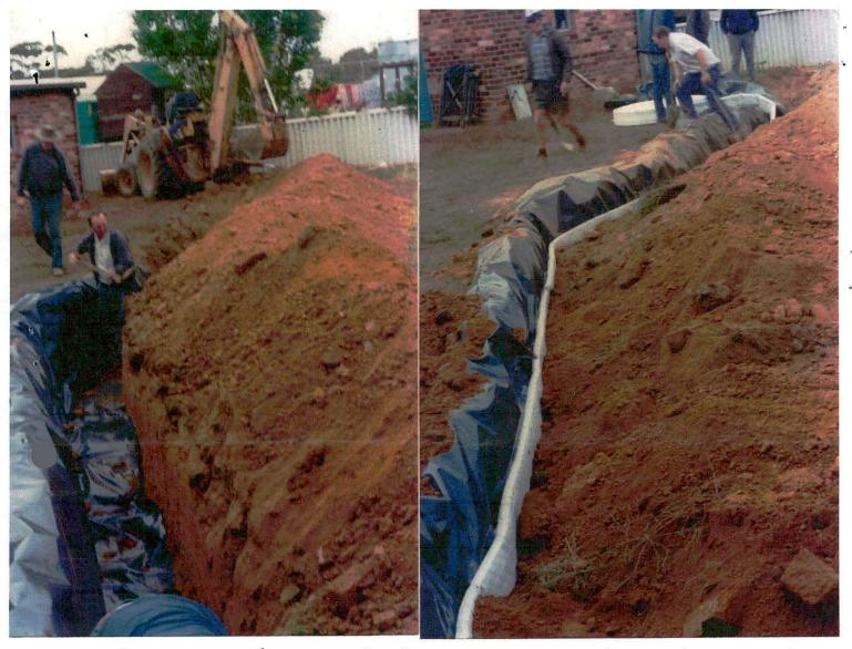
The bottom of the trench has to be on a hard bottom to seal. The strip drain works best not at the hottom. This building had wet slimy soil under the floor, walls affected (bricks and morter fretting). Twelve months later the soil was dry, wall had died out to their normal colour and no further problems and is a long term solution
