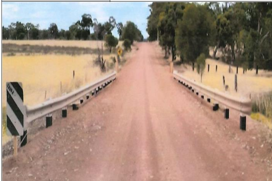
Photo abutment 1 down road
