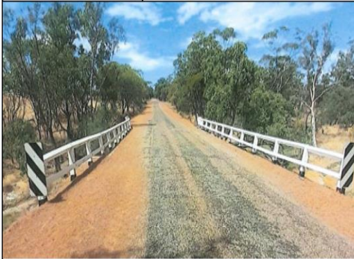
Photo abutment 1 down road
