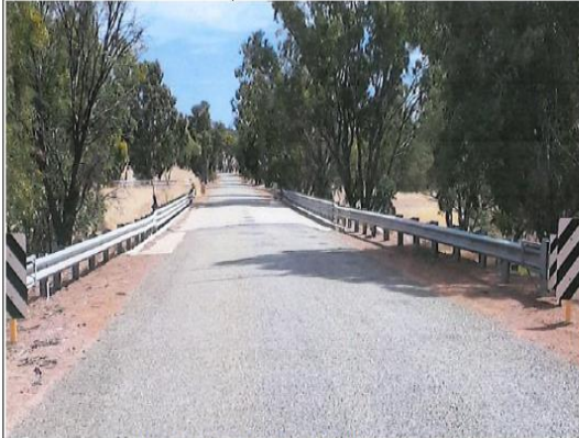
Photo abutment 1 down road
