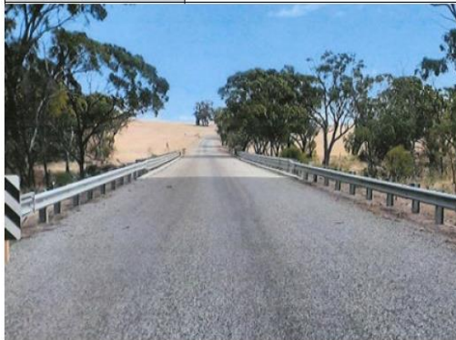
Photo abutment 1 down road
