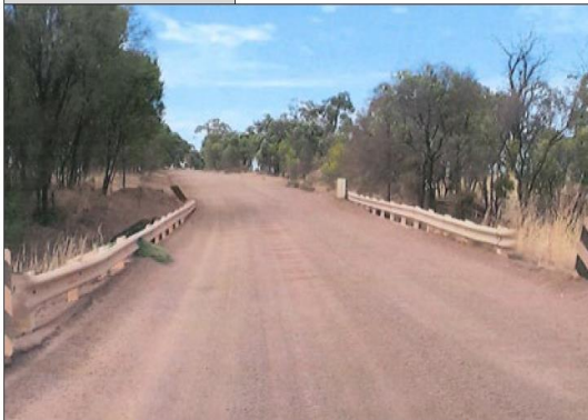
Photo abutment 1 down road
