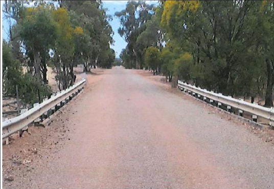
Photo abutment 1 down road
