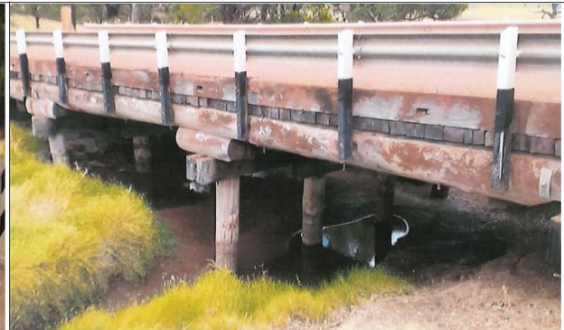
Photo left hand side from abutment 1
