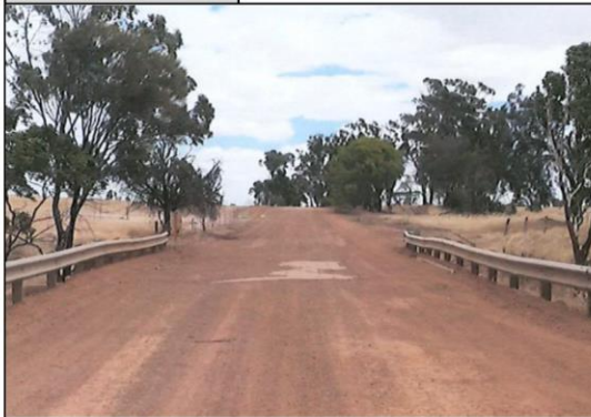
Photo abutment 1 down road
