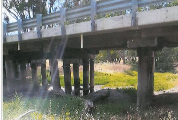
Photo left hand side from abutment 1
