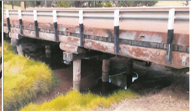
Photo left hand side from abutment 1
