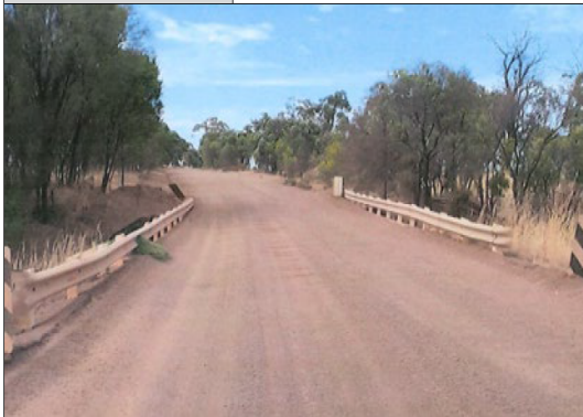
Photo abutment 1 down road
