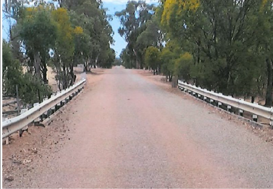
Photo abutment 1 down road
