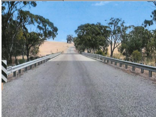
Photo abutment 1 down road
