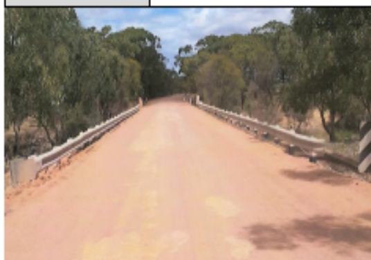
Photo abutment 1 down road
