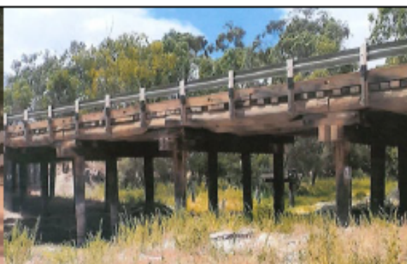
Photo left hand side from abutment 1
