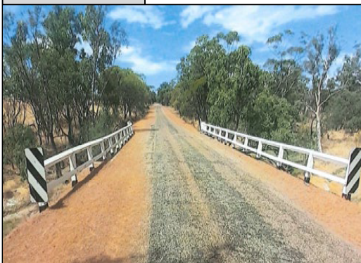
Photo abutment 1 down road
