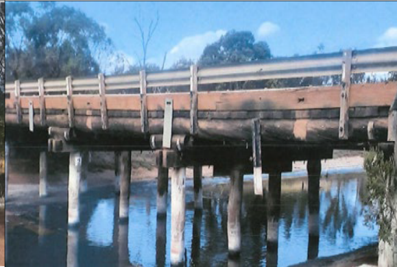
Photo left hand side from abutment 1
