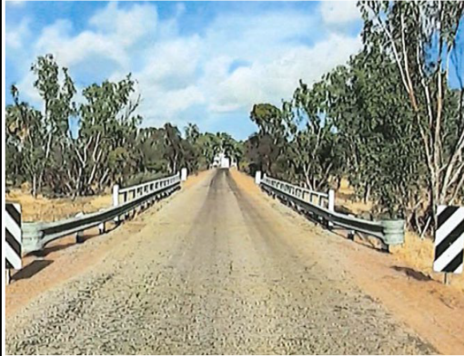
Photo abutment 1 down road
