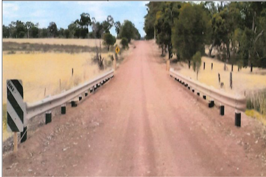
Photo abutment 1 down road
