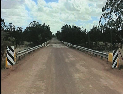
Photo abutment 1 down road
