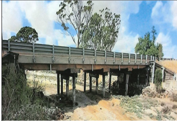
Photo right hand side from abutment 1
