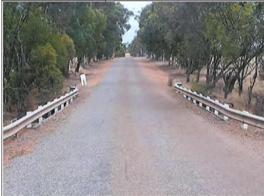
Photo abutment 1 down road
