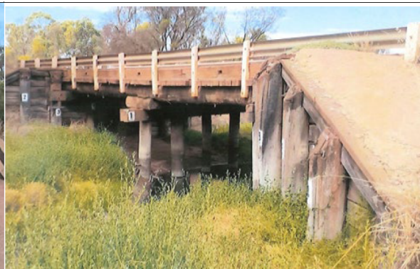
Photo left hand side from abutment 1
