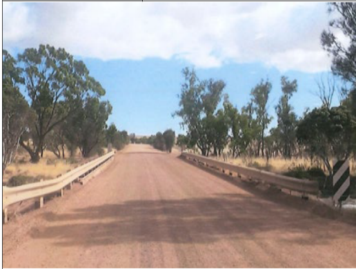
Photo abutment 1 down road
