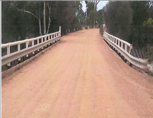
Photo abutment 1 down road
