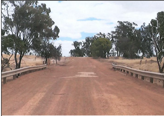
Photo abutment 1 down road
