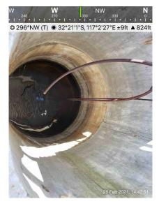
Figure 19: Photograph within the well showing the groundwater level
