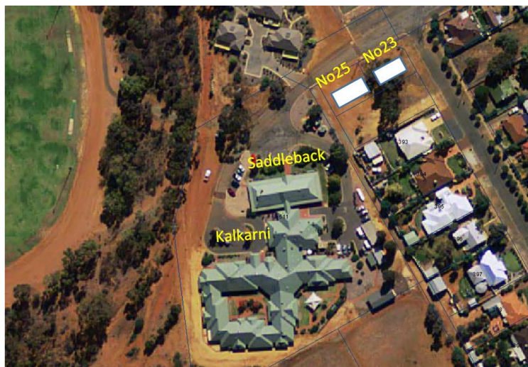
Figure 1 – Location of No.23 and No.25 Whittington Street Brookton
