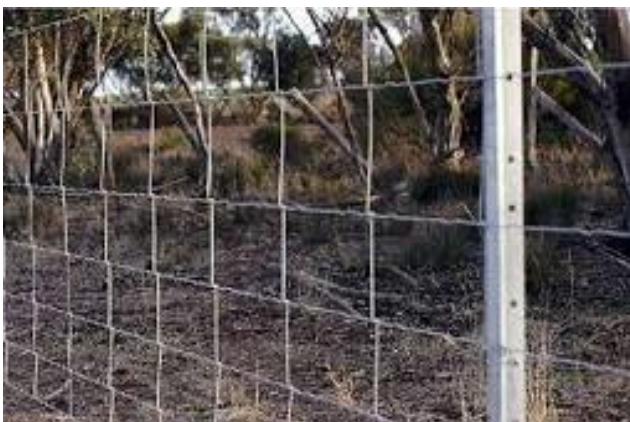
Figure 1 – Standard Ring Lock Fencing
