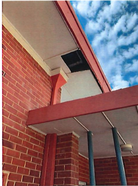
Reference picture 10: Building eaves.
