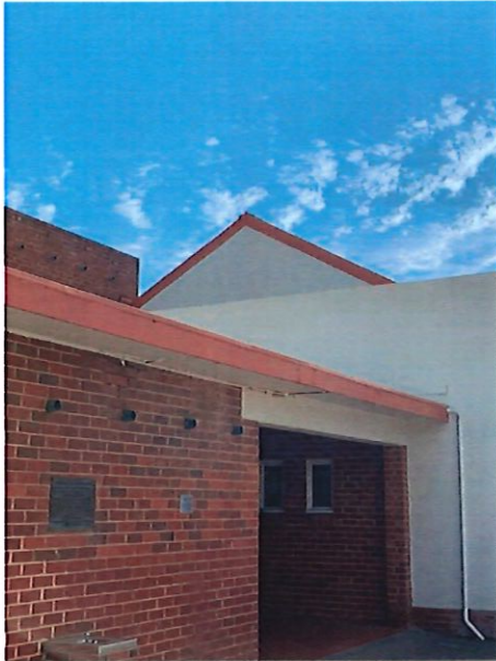
Reference picture 9: West gable end on roof.
