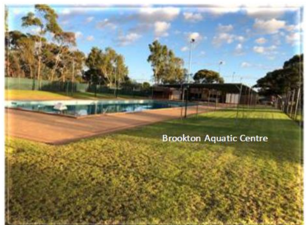
Figure 14 – Main pool and concourse looking north
