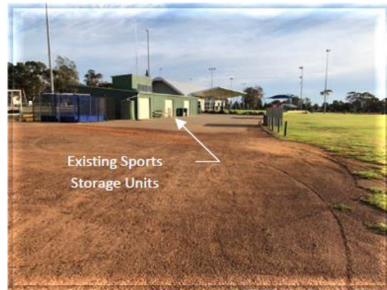
Figure 29 – Sports storage units looking north
