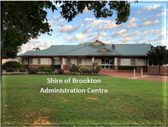
Figure 5 – Admin. Building looking north west
