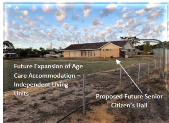
Figure 53 – Expansion area looking east
