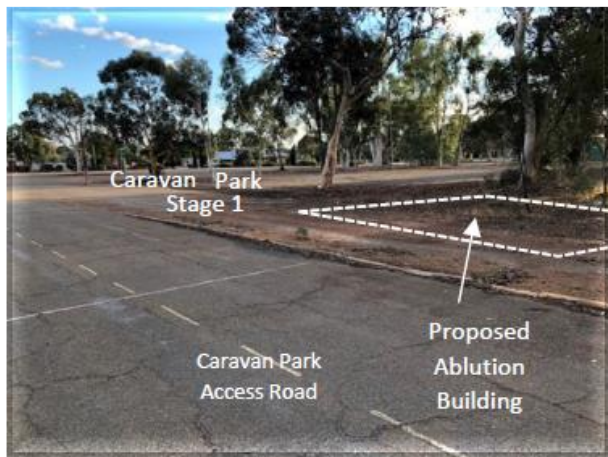
Figure 23 – Internal access road looking north
