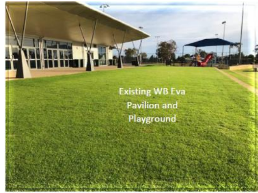
Figure 27 – WB Eva building Looking north
